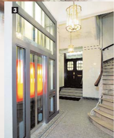
Poststraße: 3 Modernised passenger elevator with glass housing in an art nouveau building.
