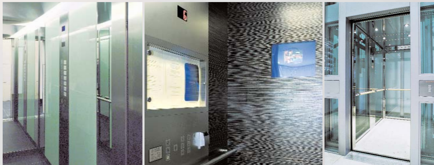
Alsterhaus: 1 Modern car with raised frosted glass, mirror panels and a natural stone floor.
